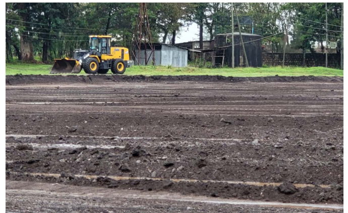
The soccer field under construction
